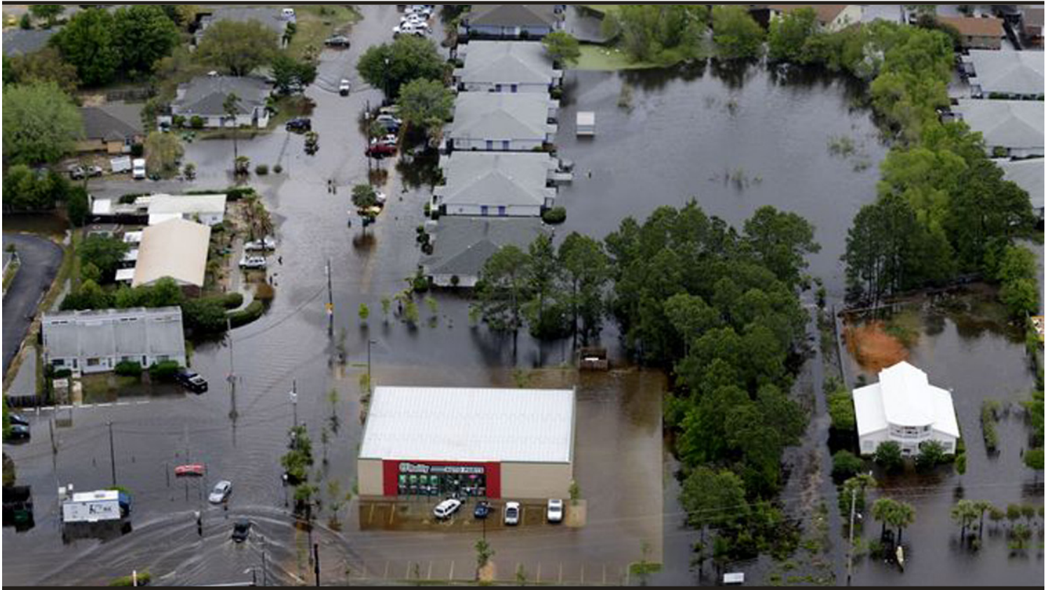
Floods ravaged the Gulf Breeze area in the Florida Panhandle as a result of severe storms in April 2014. (Photo by Katie King, kking@pnj.com. Copyright 2014.)
