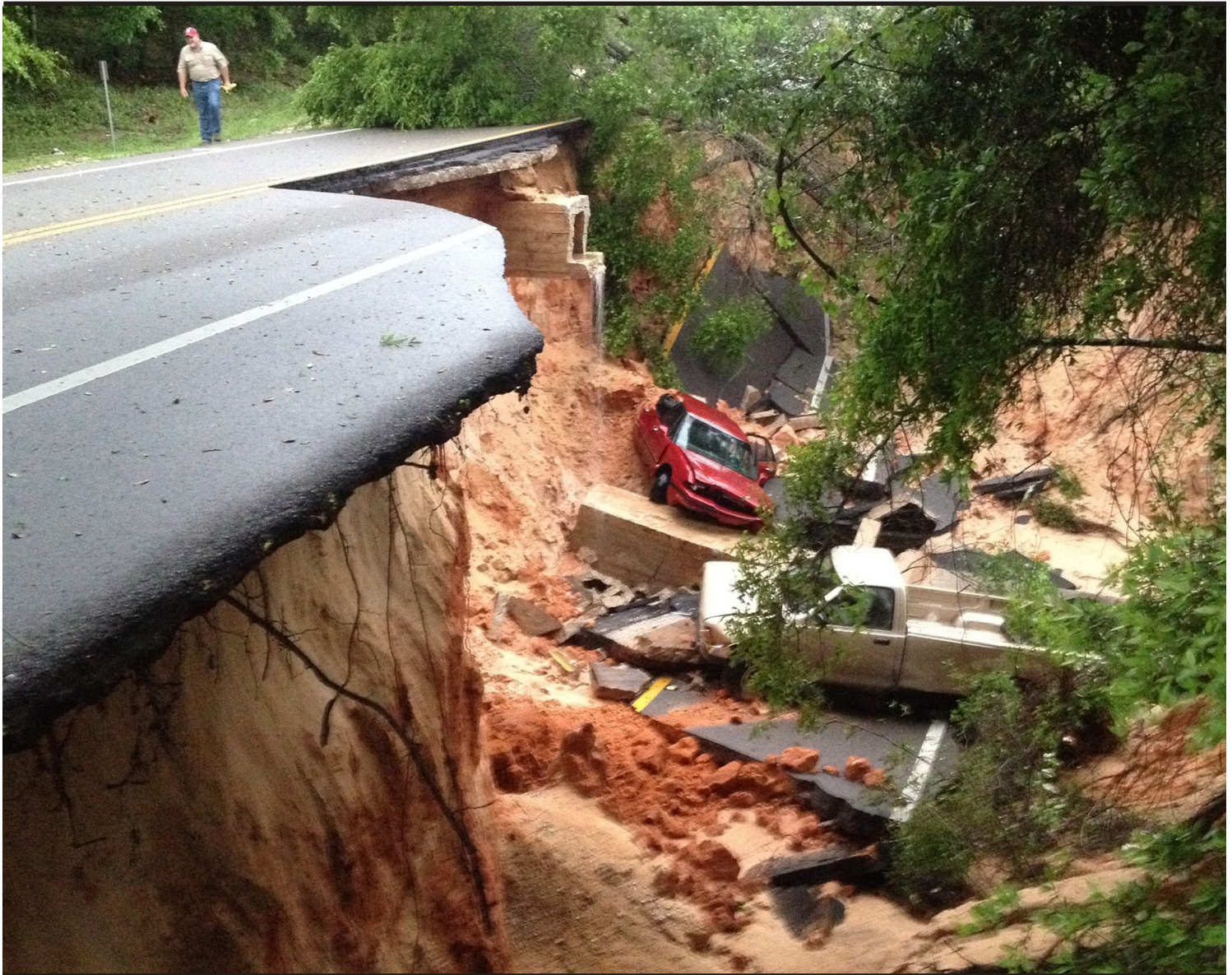
As a result of heavy rainstorms in April 2014, Scenic Highway collapsed into the bay, sending at least two trucks plummeting approximately 40 feet. The Army Corps of Engineers initiated emergency permitting procedures to aid in repair of infrastructure. Scenic Highway is expected to reopen at the end of June. (Photo by Katie King, kking@pnj.com. Copyright 2014.)
