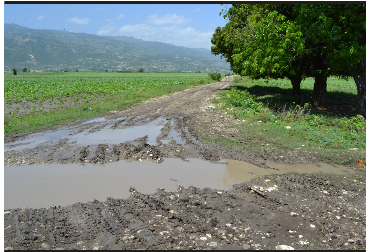
Campeche, a rural road in the Cul-de-Sac region of Haiti. Earthen and rock road surfaces are easily overcome by local drainage ways in low-lying areas. This example of a known water crossing will require a proposed drainage feature, most likely a ford, as part of the improvements to manage the water flowing through this area. (Photo by Crystal Markley)
