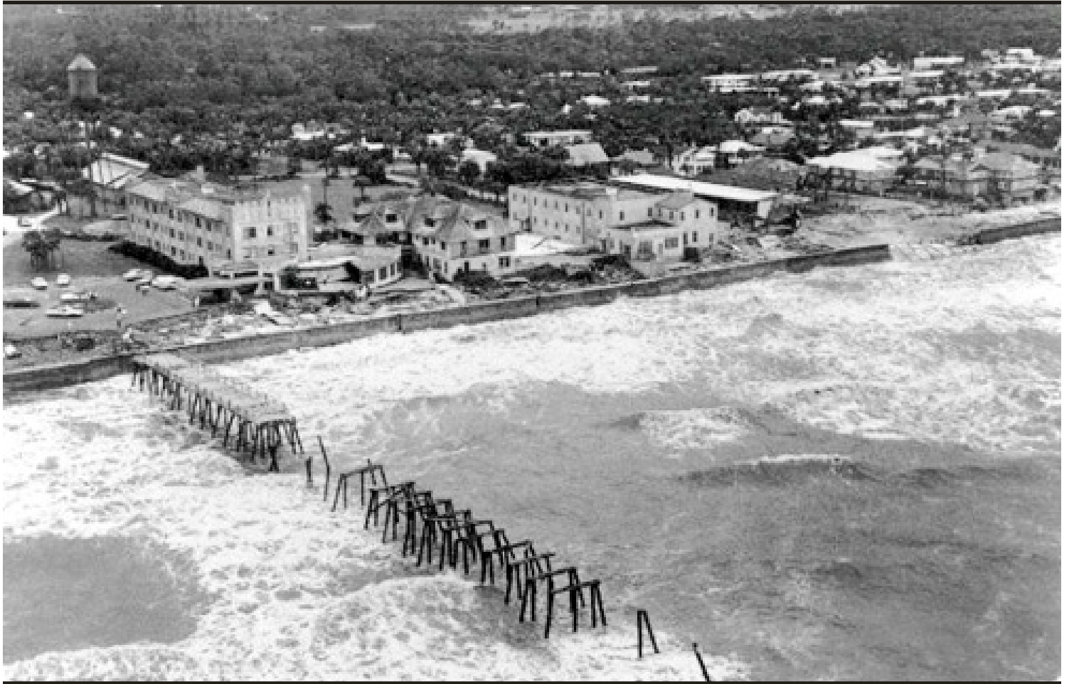
The Atlantic Beach Hotel and pier were devastated by the impacts of Hurricane Dora. The storm lingered off the Atlantic coast for nearly 24 hours, allowing winds to drive the storm surge to a point 10 feet above normal tide. (Photo courtesy of Jacksonville Historical Society)
