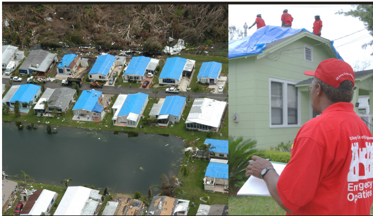
A bird's eye view of Port Charlotte, which was severely impacted by Hurricane Charley, one of four major storms to strike Florida during the 2004 Atlantic hurricane season. When conditions warrant, Operation Blue Roof provides temporary roof coverings until permanent repairs can be made. (USACE file photo)
