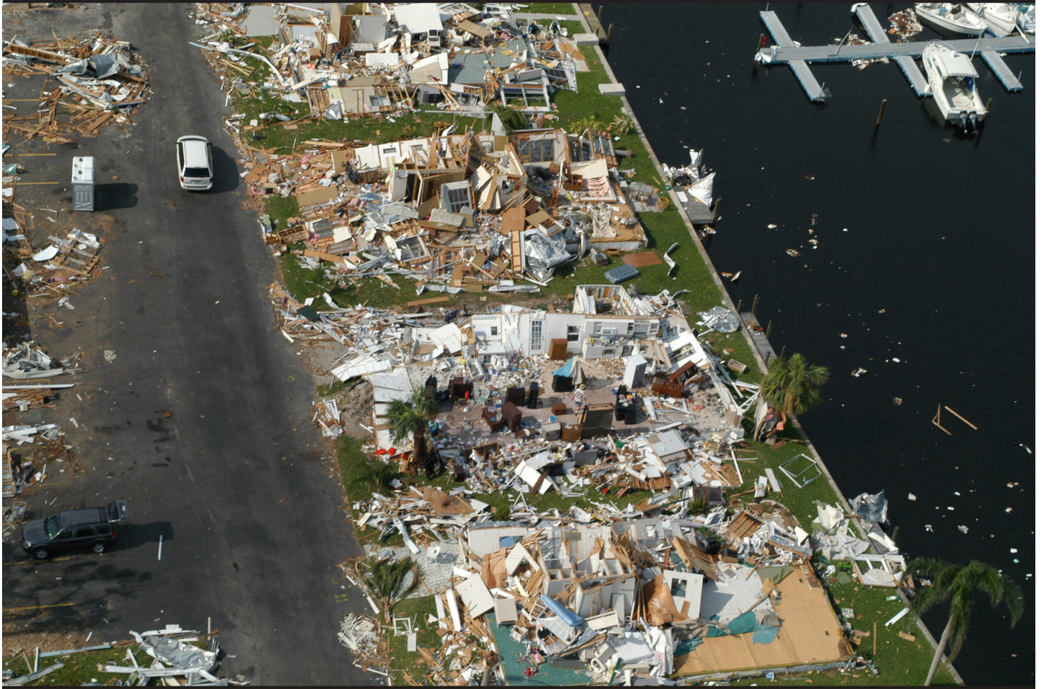
Hurricane Charley caused widespread damage to homes and businesses in southwest Florida when it came ashore near Port Charlotte Friday, August 13, 2004. Charley was one of four hurricanes that hit the state that year. (USACE file photo)
