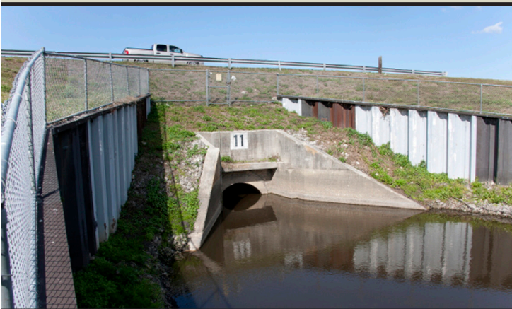
Culvert 11 before removal in March 2012. (USACE file photo)
