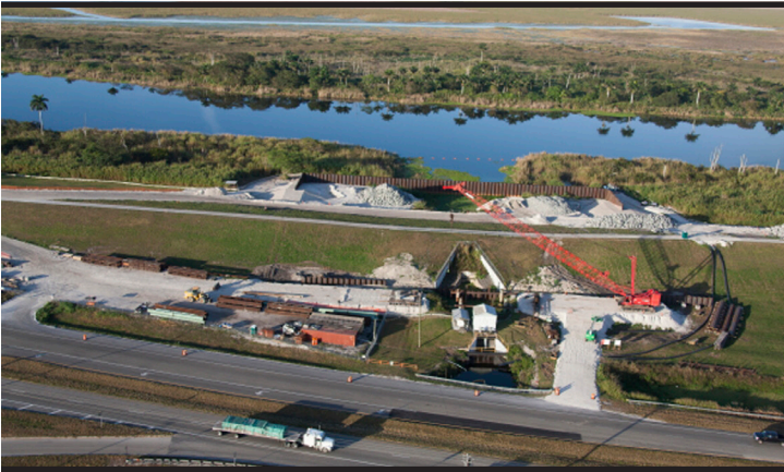
With traffic from U.S. 27 in the foreground, crews work on installing a temporary cofferdam at the Culvert 4A site near South Bay in December. The cofferdam, which must be robust enough to hold back Lake Okeechobee should it start rising, must be in place before the old culvert can be removed. (USACE photo)
