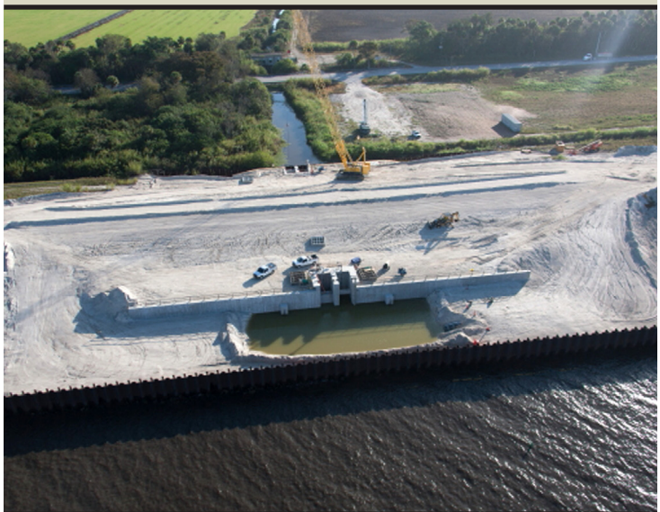
Culvert 11 nearing completion in December 2013. (USACE file photo)
