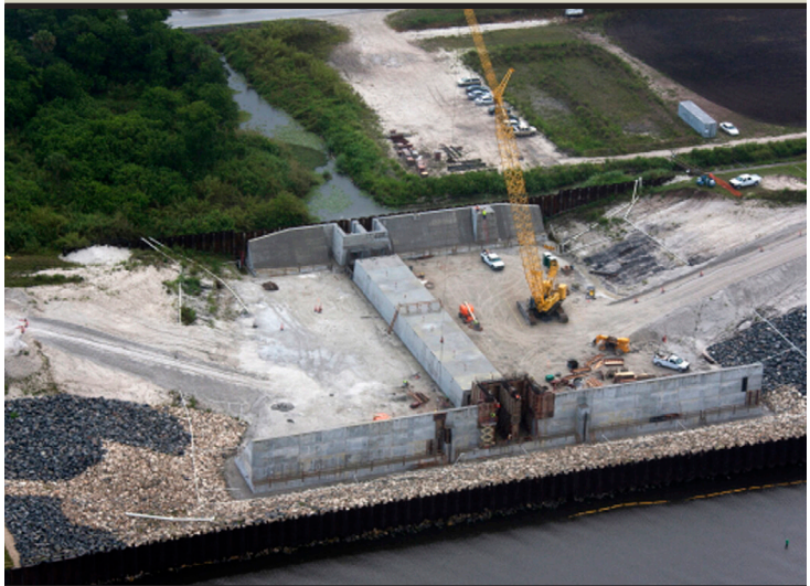
The replacement structure begins to take shape in April 2013. (USACE file photo)
