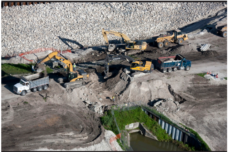
Removal of Culvert 11 in July 2012. (USACE file photo)
