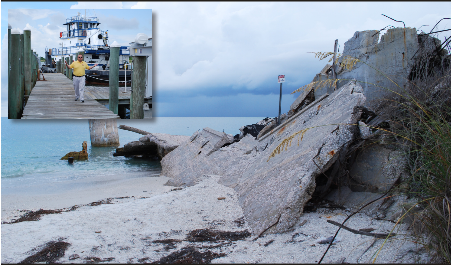
Storm surge and wave erosion destroyed portions of Fort Dade's artillery battery on the northern point of Egmont Key. Inset: Project Manager Milan Mora isn't telling a fish tale, he's signaling to a group of Corps and NOAA Fisheries team members that he's ready to move out on a tour of Egmont Key.
