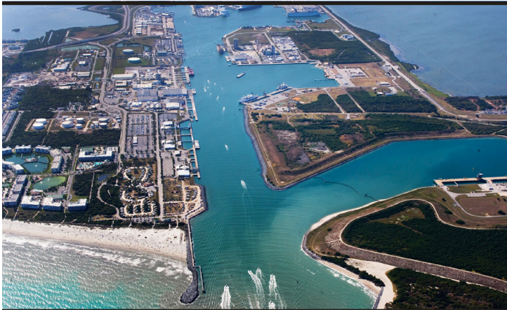
The Canaveral Harbor deepening project will improve navigation safety and allow passage of larger ships. (USACE file photo)
