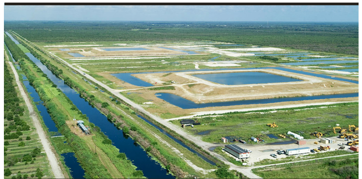
Pictured here is a test cell for the Caloosahatchee River (C-43) West Basin Storage Reservoir Project. The project will capture and store basin stormwater runoff, along with a portion of water discharged from Lake Okeechobee, before release into the Caloosahatchee River. (Photo by Patrick Lynch, South Florida Water Management District)
