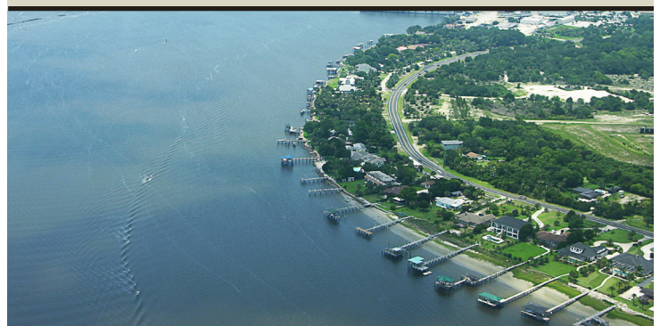
Jacksonville Harbor’s Mile Point Project will improve navigation safety by reducing the impacts of ebb tide crosscurrents at the confluence of the St. Johns River with the Intracoastal Waterway. (USACE file photo)
