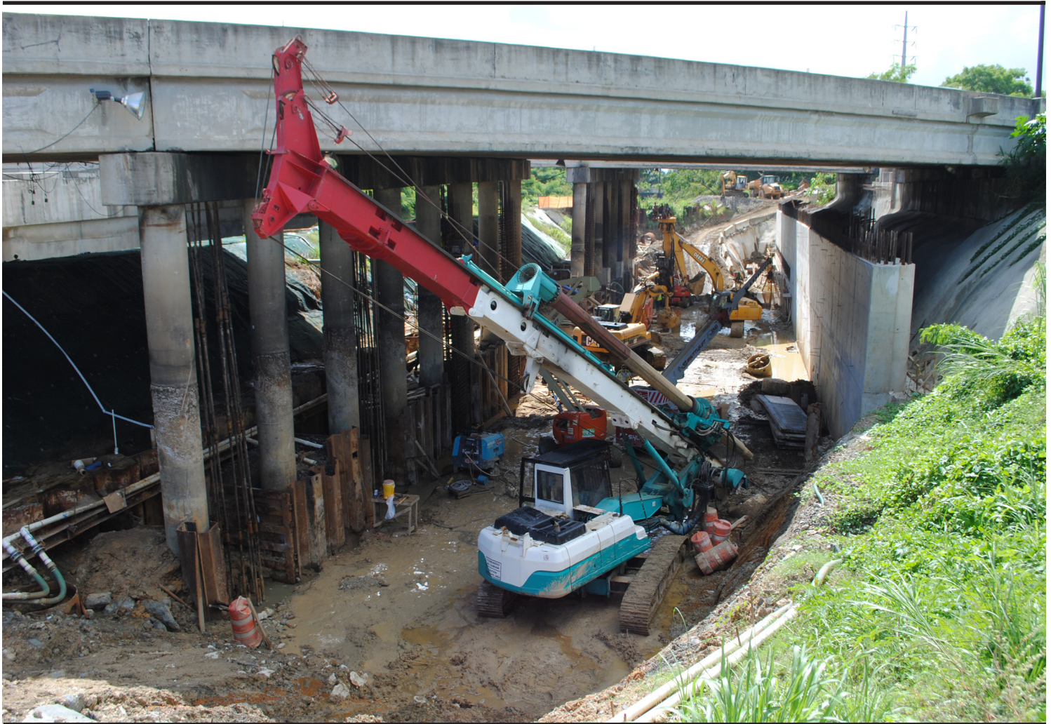
Crews work on the De Diego bridge in San Juan, Puerto Rico as part of the Rio Puerto Nuevo flood control project. The contract is one of 100 contract awards worth a combined $1.6 billion that's being overseen by the Jacksonville District Construction Division. (Photo by John Campbell)
