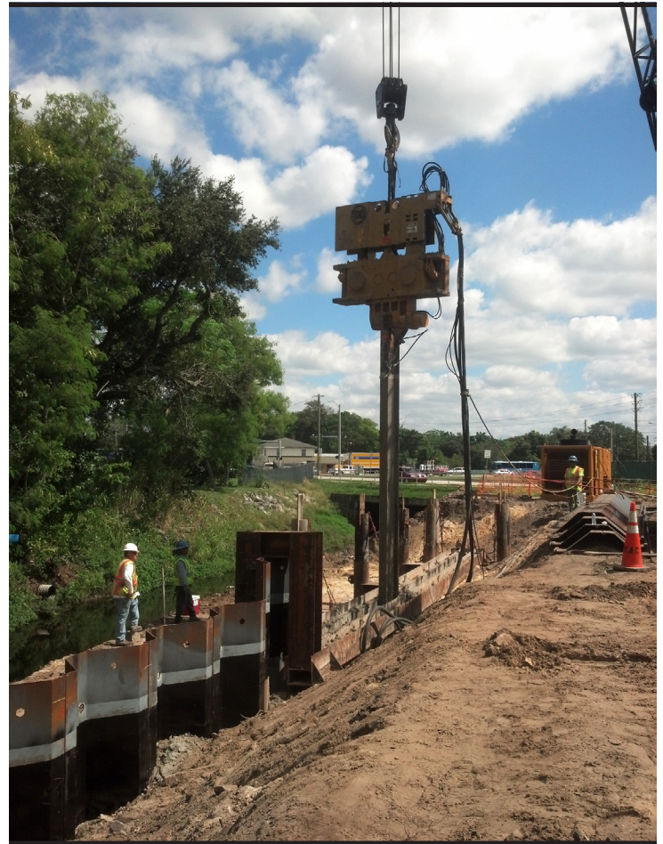
At the Wares Creek Flood Control Project in Bradenton, Fla., crews prepare for the installation of sheet pile, using a chisel beam to penetrate the dense limestone layer below. Each of three phases of the project was awarded to an 8(a) small business firm. (Photo by Jean Wilson)
