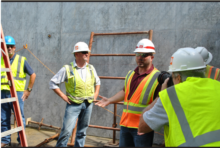
Always make sure everyone on site is wearing the appropriate personal protective equipment (PPE), even those who do not intend to be on camera. (Photo by Jenn Miller)
