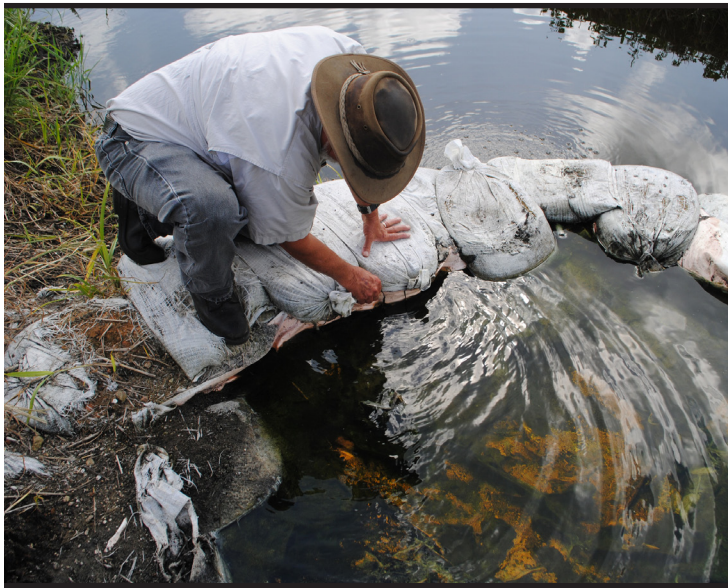
Calvin Grinslade, civil engineering technician with the South Florida Operations Office, takes a close look at a seepage site on the Herbert Hoover Dike as part of the weekly inspections on the earthen structure surrounding Lake Okeechobee. The Operations Division conducted weekly inspections as part of its response to elevated water levels in the lake due to heavy rain this summer. (Photo by John Campbell)
