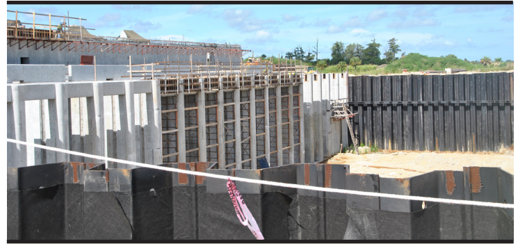
The Faka Union Pump Station is one of three pump stations for the Picayune Strand Restoration project. The construction contract for Miller Pump Station, the third and final pump station, was awarded in September. Faka Union is scheduled to be completed in fall 2014. (Photo by Jenn Miller)
