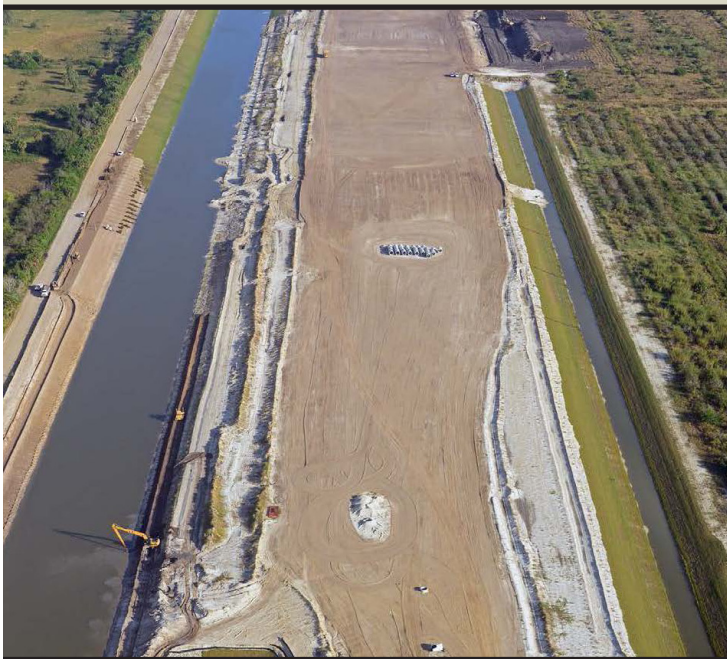
An intake canal was excavated and sodded as part of the ongoing construction at the C-44 Reservoir and Stormwater Treatment Area project near Indiantown in Martin County, Fla. (Photo courtesy of Phillips & Jordan, Inc.)
