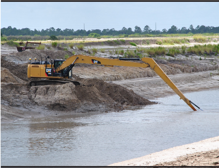
A contractor works in the intake canal as part of the C-44 Reservoir and Stormwater Treatment Area project near Indiantown in Martin County, Fla. The Jacksonville District Construction Division placed $385 million of work during fiscal Year 2013, and leaders expect a bigger year in 2014. (Photo by Jenn Miller)
