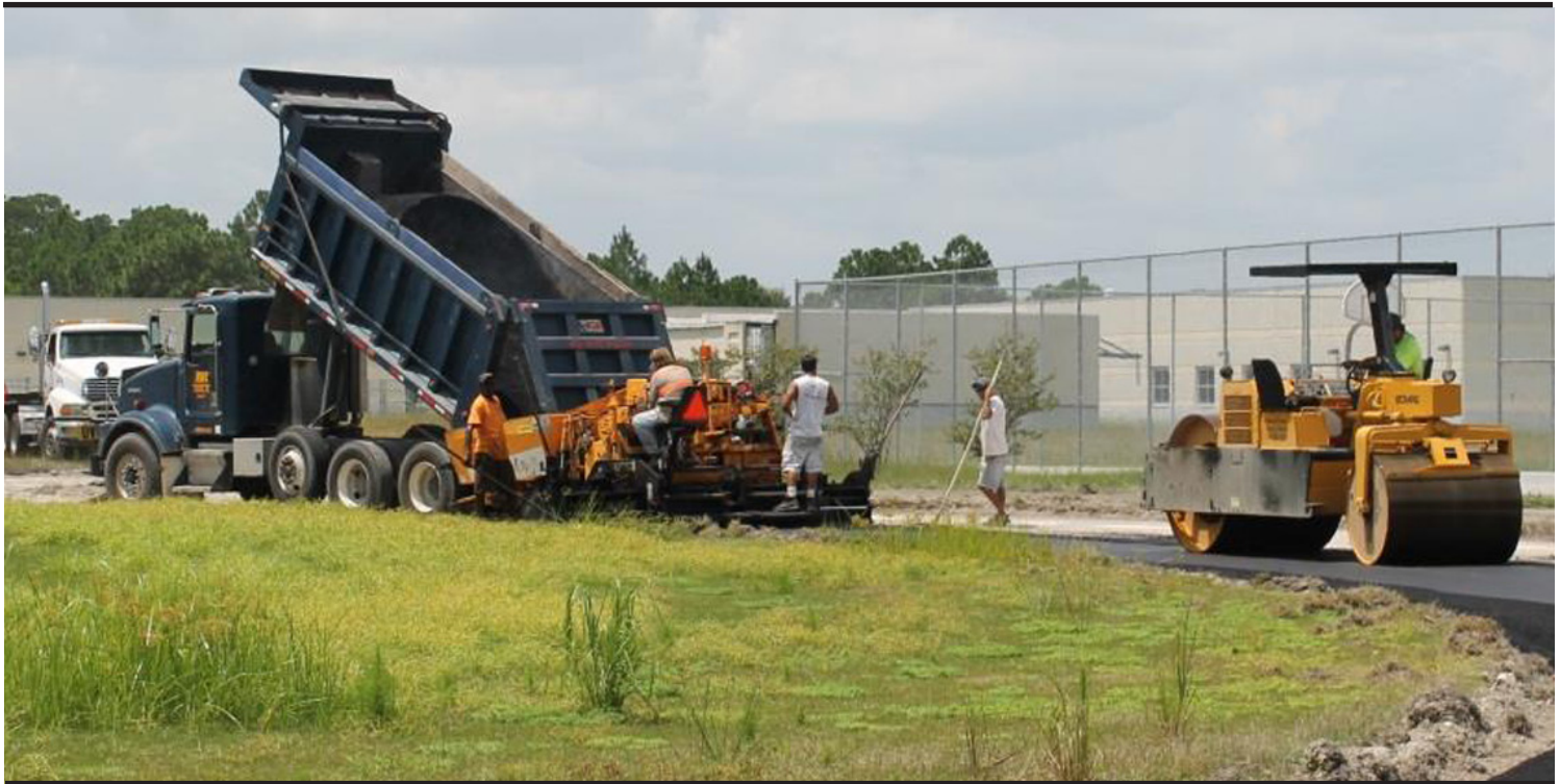
Crews install a new athletic track at Odyssey Middle School in Orlando, Fla. following completion of remedial actions for the Pinecastle Jeep Range Formerly Used Defense Site. (Photo courtesy of ITSI Gilbane)
