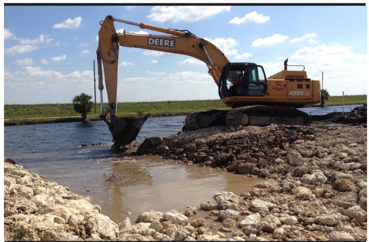
The old Tamiami Trail roadway was broken through May 15 during roadway removal efforts, as part of the Tamiami Trail Modifications project in Miami, Fla. (Photo by Chris Rego)
