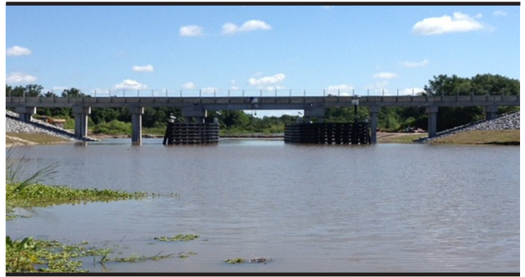
Water is now flowing beneath the newly constructed CSX Railroad Bridge after the northern earthen plug was removed at the Kissimmee River Restoration (KRR) project May 8. (Photo by Erin Duffy)
