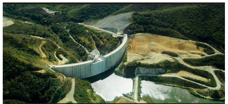
The backside of Portugués Dam as water begins to collect in the reservoir. Initial filling began on June 16 with a level of 372 feet, and will continue until it reaches 439.8 feet, its maximum normal operating level. (USACE file photo)
