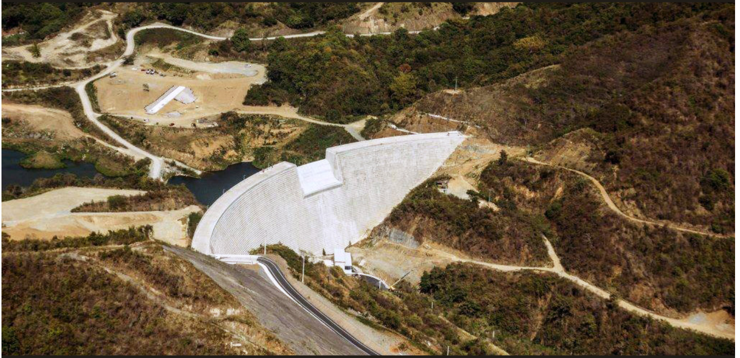
Portugués Dam in Ponce in southern Puerto Rico was dedicated in February 2014. Jacksonville District closed outlets on the 220-foot structure in mid-June to begin filling the reservoir. (USACE file photo)
