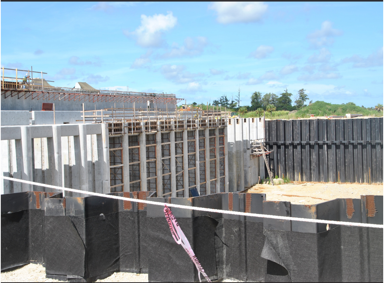
The Faka Union Pump Station is scheduled to be completed in fall 2014. (Photo by Jenn Miller)
