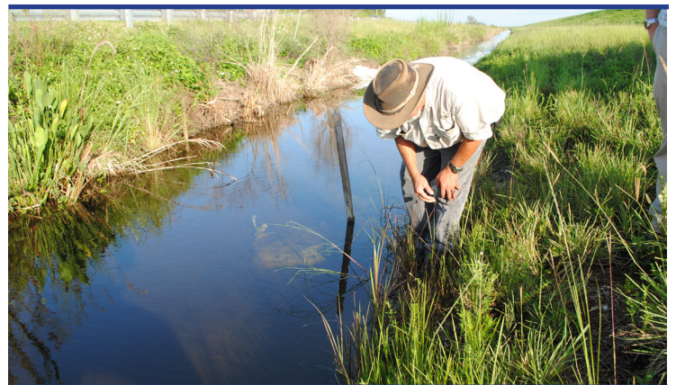
Calvin Grinslade, civil engineering technician with the South Florida Operations Office, takes a close look at the toe ditch near Herbert Hoover Dike as part of the weekly inspections conducted this summer on the earthen structure surrounding Lake Okeechobee. The intent of the inspections is to identify minor issues and address them before they turn into major problems. (Photo by John Campbell)
