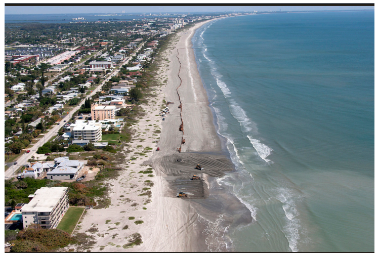
Contractors pump sand onto miles of Brevard County beaches. (USACE file photo)
