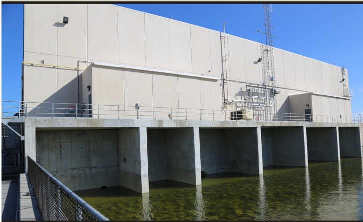
Construction was completed on the Picayune Strand Restoration project's Meritt Pump Station in October. The pump station is a key piece of infrastructure for the Picayune Strand Restoration Project that will aid in the restoration of more than 55,000 acres of natural habitat. (Photo by Ty Erickson)
