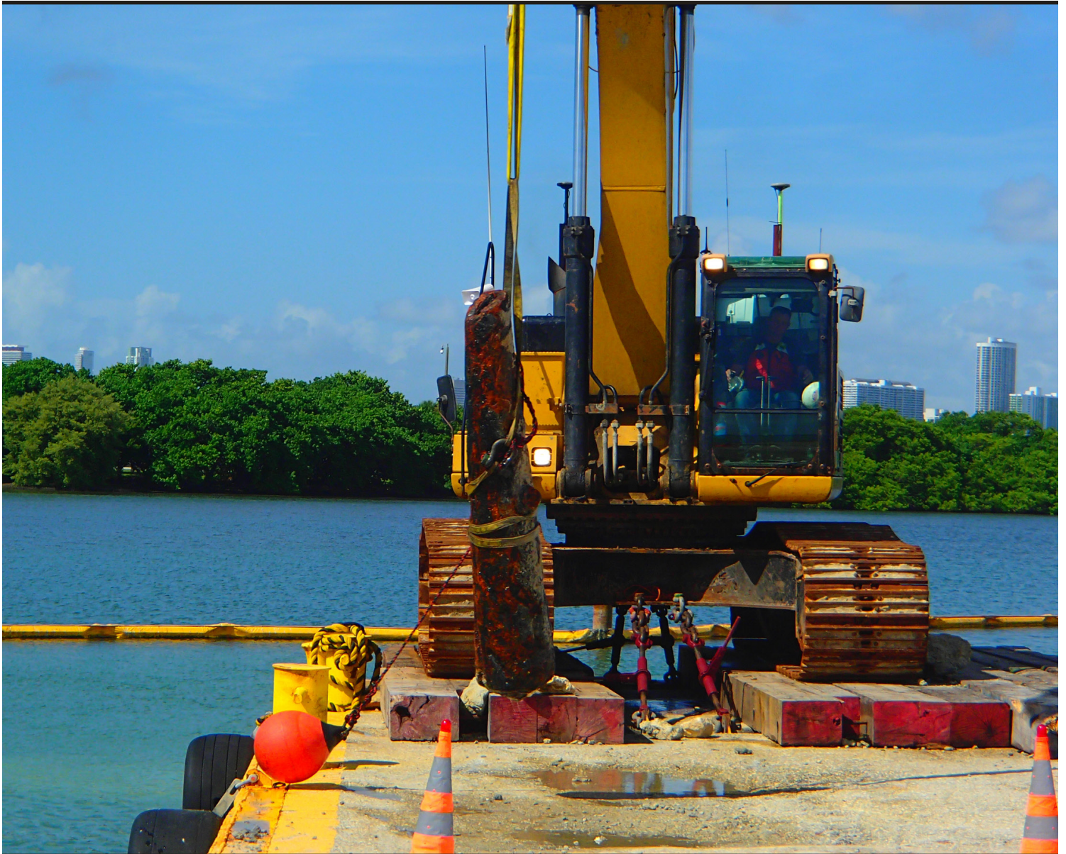
A GLD&D employee slowly lowers an early 18th century cannon onto a dock, readying it for inspection and transport. (Photo by Grady Caulk, USACE)
