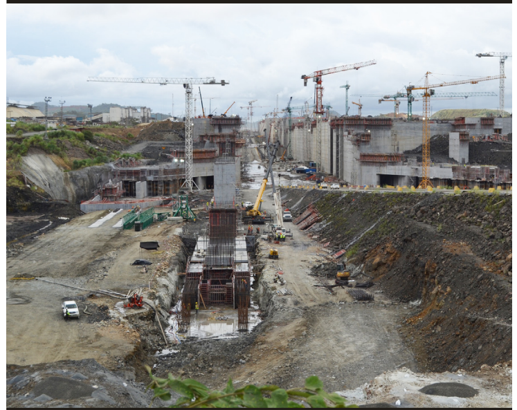
Current construction being performed on the Panama Canal. Tours were given of the canal as the American Society of Civil Engineers (ASCE) celebrated the Panama Canal's 100th Anniversary. Maj. Gen. (Ret.) Meredith W. B. Temple, P.E. PMP, F.ASCE, told those attending the conference what engineers can learn from the enormity of the original Panama Canal project, the design and building of it and the challenges that the initial builders faced. (USACE file photo)
