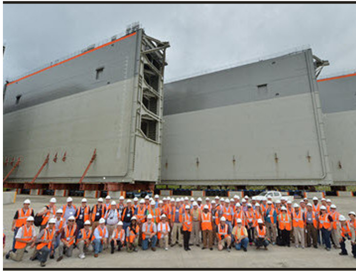
A group of attendees at ASCE's Global Engineering Conference in Panama tour the Atlantic Third Lane Bridge and Lock canal expansion project, gathering at a temporary dock where new lock gates await installation. (Photo by Panama Canal Authority)
