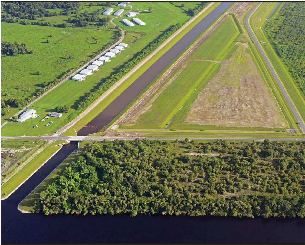
Construction was completed on the first construction contract for the Indian River Lagoon-South's C-44 Reservoir and Stormwater Treatment Area in July. The contract included construction of approx. 7 miles of canals, access roads, staging areas, and other pieces of infrastructure needed to move forward with the larger components of the project. (Photo by Phillips & Jordan, Inc.)
