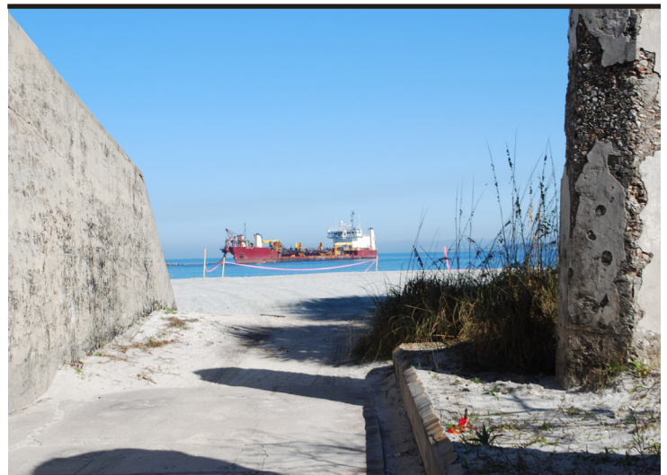
Dredged material from Tampa Harbor maintenance is beneficially used on Egmont Key, which is severely eroding. The sand placement will help protect cultural resources on the island. (USACE file photo)
