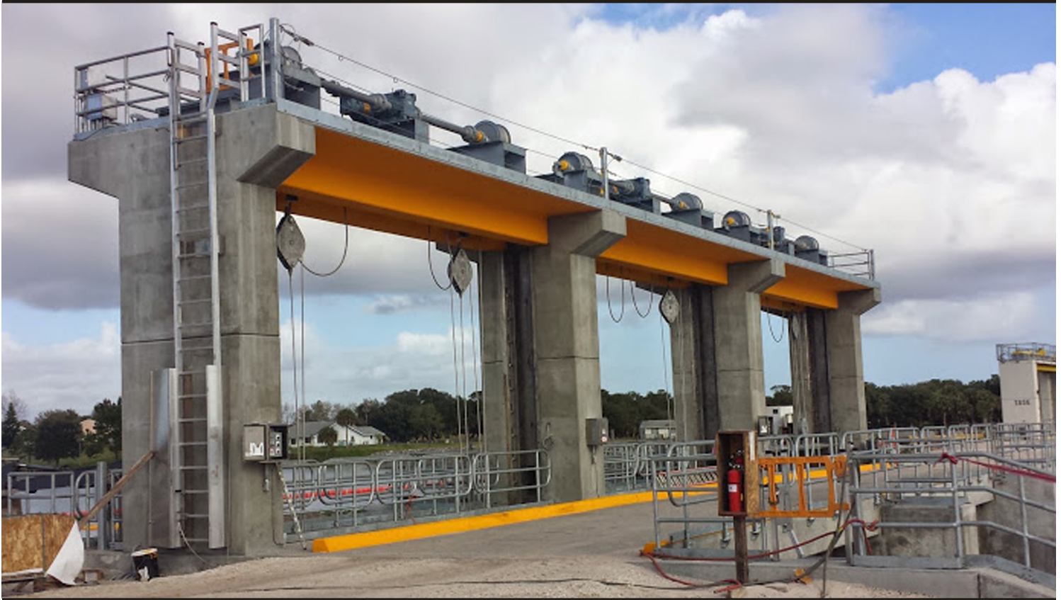
Construction continues at the S-65EX1 Gated Spillway, part of the Kissimmee River Restoration project. The structure will enable water managers to maintain river stages during extreme rain events to provide authorized flood protection to those who may be impacted by extreme rain events in the area. (USACE file photo)
