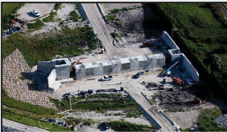
Culvert 13 (S-272) - Reconstruction
