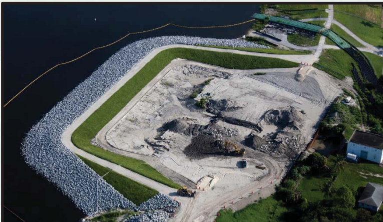
Culvert 12 (S-275) - Excavation
