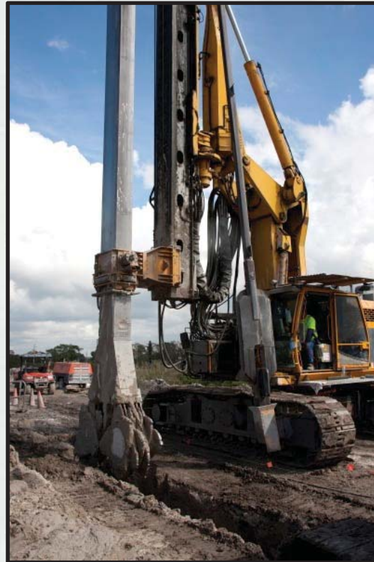
Cutter Soil Mixer (CSM)
