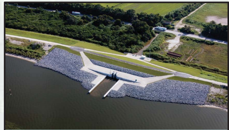
Culvert 11 (S-269) - Completion
