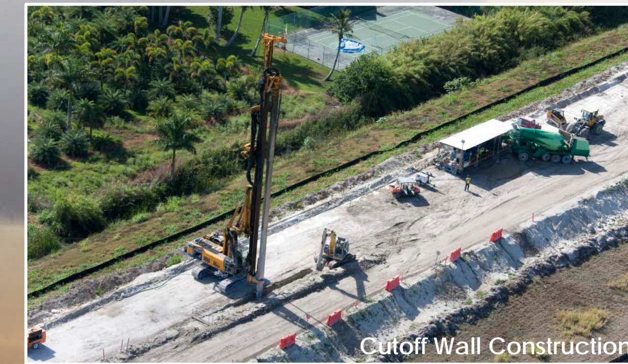
Cutoff Wall Construction
