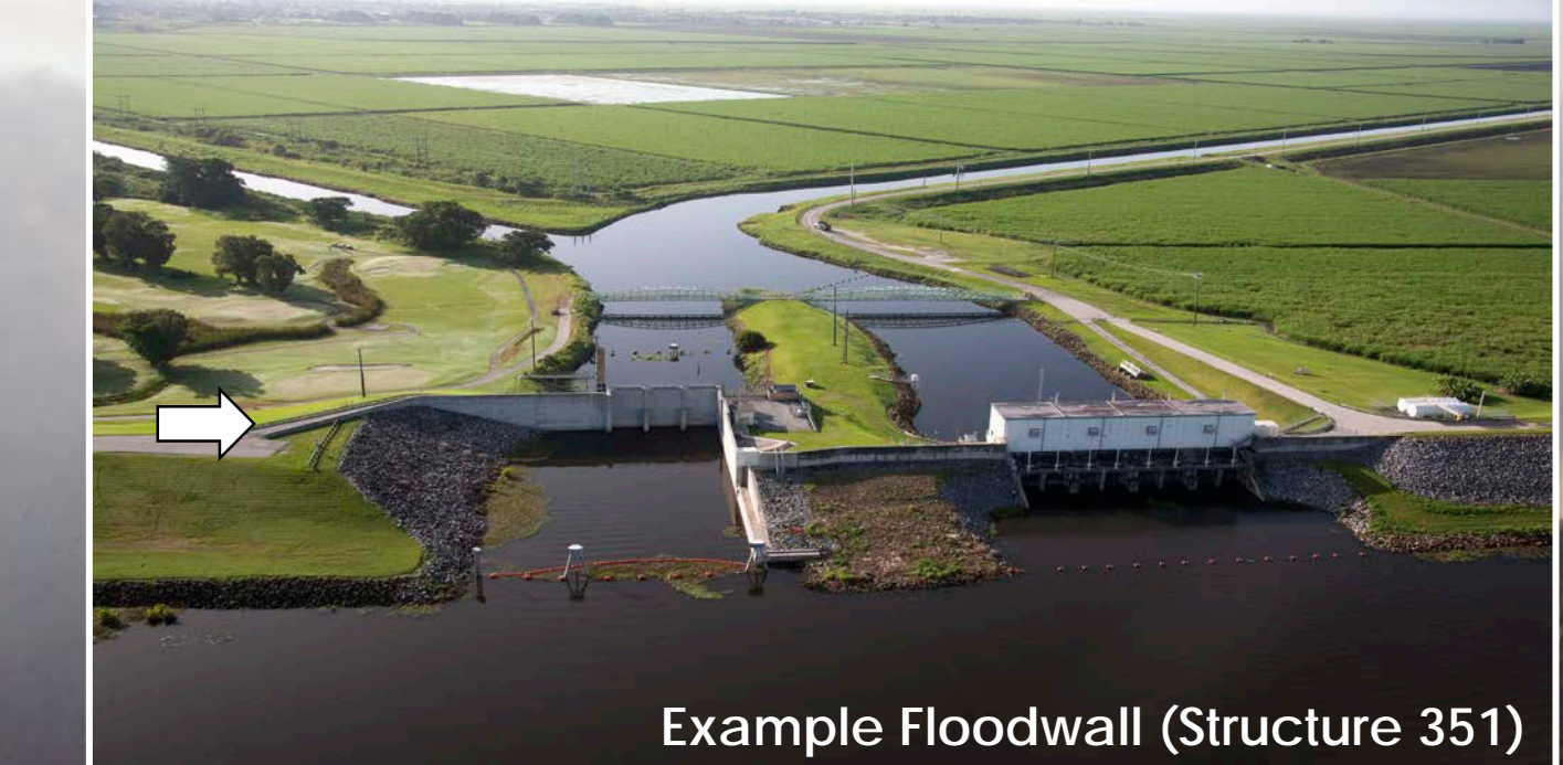
Example Floodwall (Structure 351)
