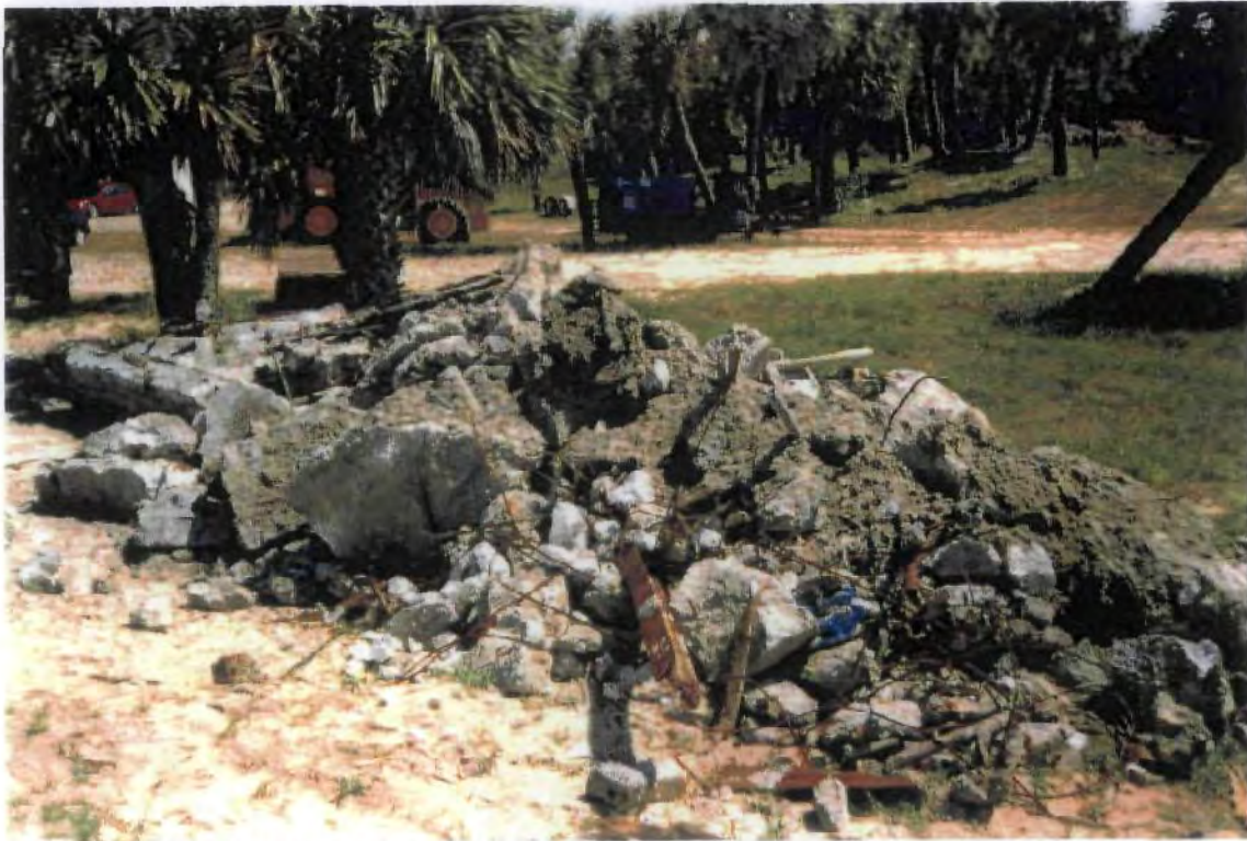
Typical mixed debris ready to be loaded into dumpsters for disposal.
