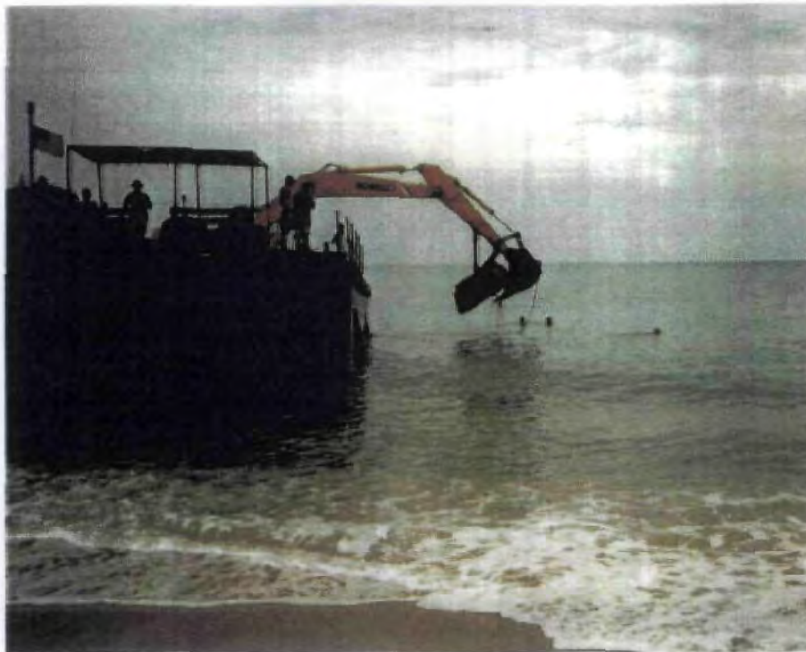
Track hoe lifting a type IV scully from the water with the bucket. Note the three divers in the water beyond the trackhoe arm.
