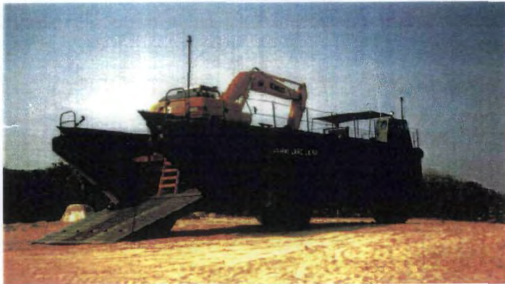
LARC 52 with trackhoe mounted inside well deck
