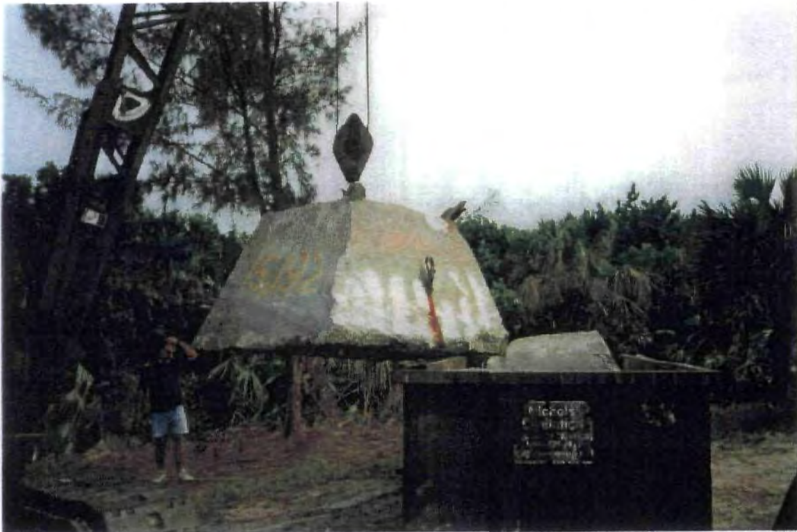
Scully being loaded into dumpster for disposal. Note the weight of scully painted on side (15,192 lbs.).
