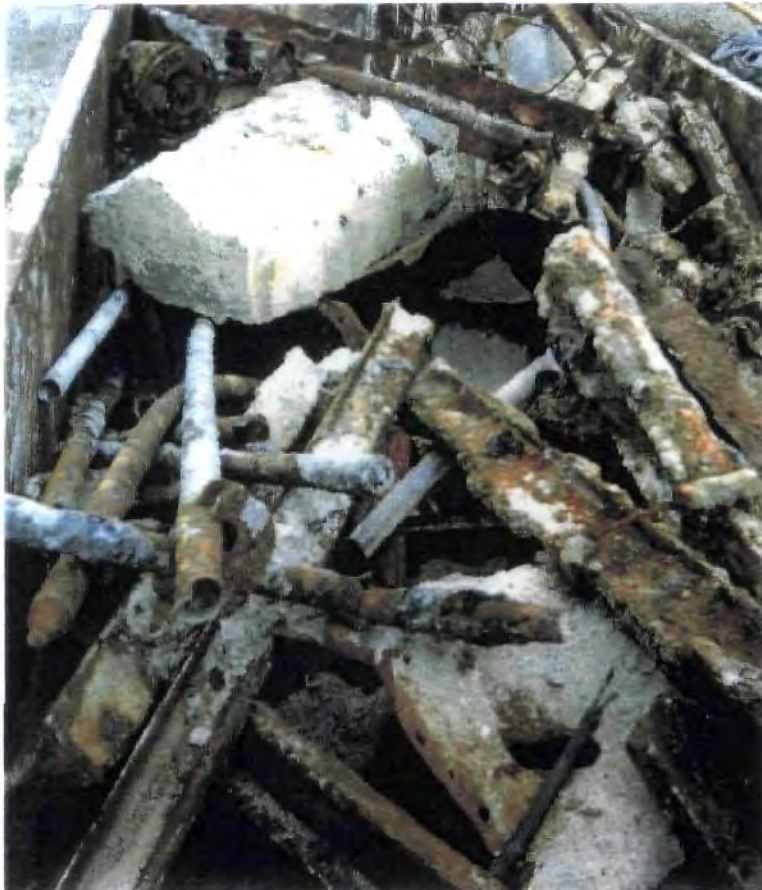
Typical metal debris (railroad irons and tubular scaffolding pipes ) and concrete debris loaded in Dumpster for disposal.
