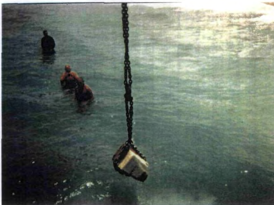
Type I scully being lifted from the water with chain rigging.
