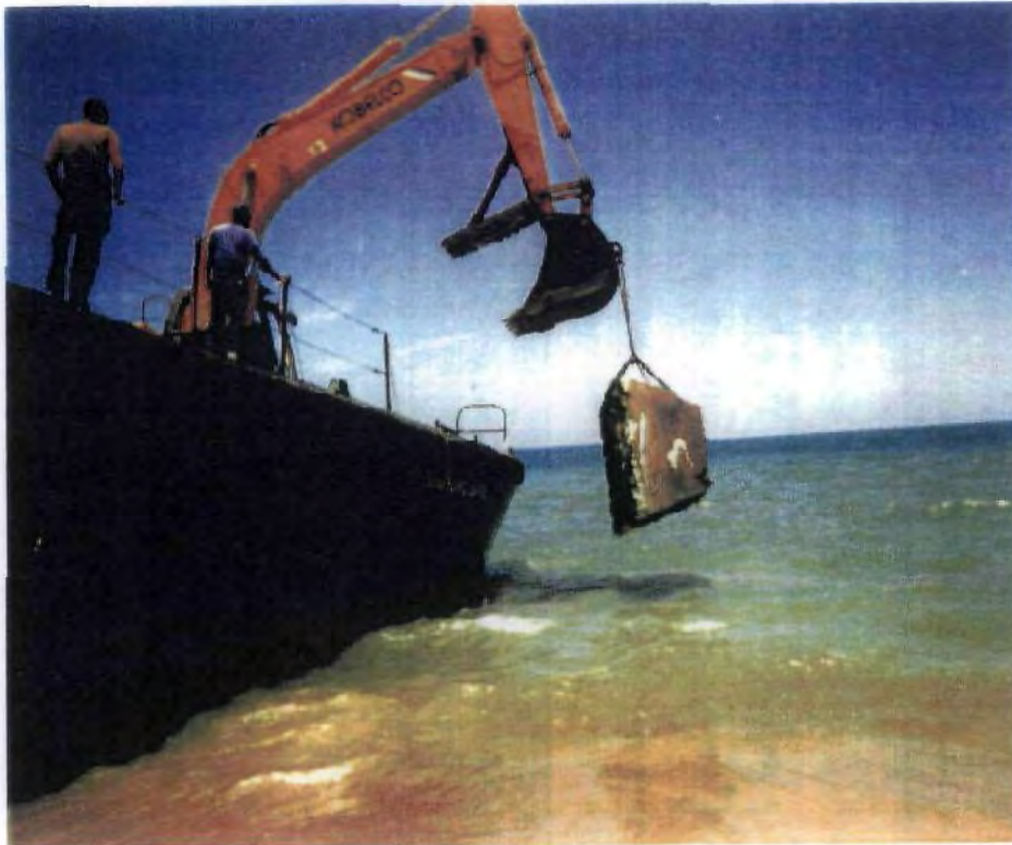
Track hoe lifting a type IV scully from the water with chain rigging.
