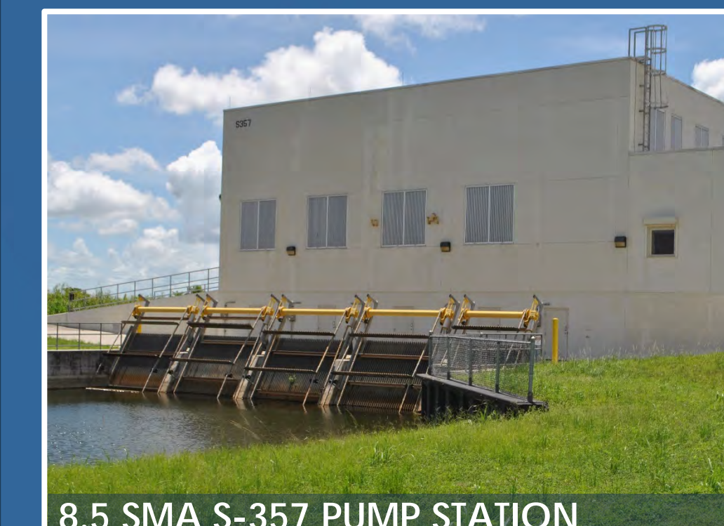
8.5 SMA S-357 PUMP STATION
