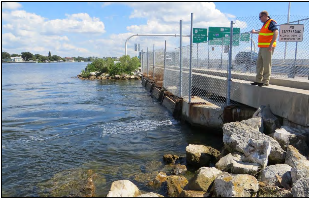
Figure 1-2 Tide flap gates at incoming (high) tide.
