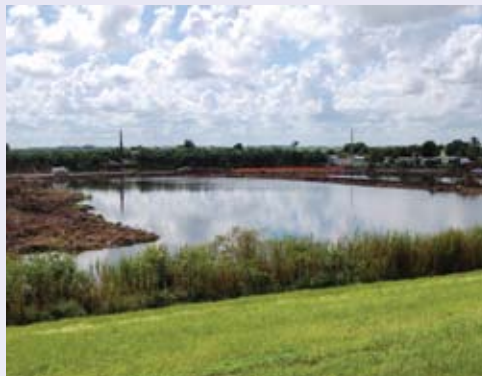
These quarries will be filled by this spring to benefit the dike, which is pictured in the foreground.
